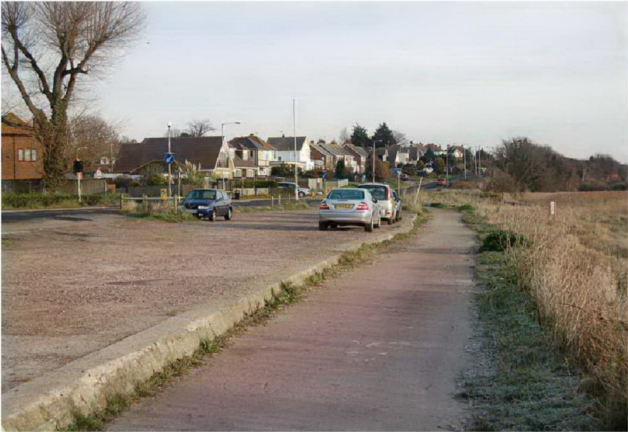
Site of proposed flood wall – (on landward side of informal car park)
